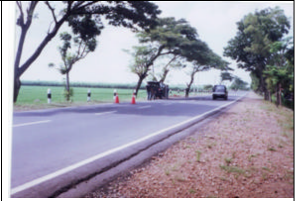
Ruas Jalan Caruban-Ngawi Km Sby 154+130
