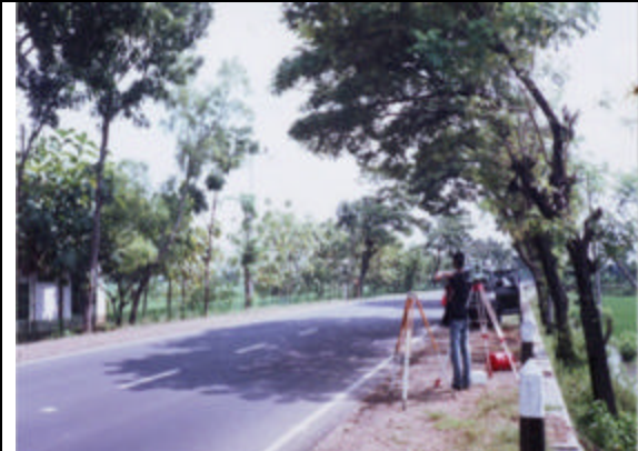
Ruas Jalan Caruban-Ngawi Km Sby 154+130
