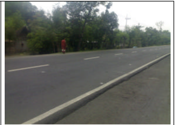
Ruas Jalan Caruban-Ngawi Km Sby 153+750
